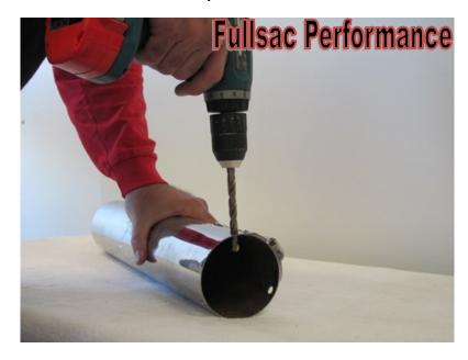
**Step 4** -Starting with the 1/8 drill bit, drill through your center punch marks. If your marks are not perfectly centered, angle the drill to correct this. Next drill through with a ¼ inch drill and then a 3/8 inch drill.
